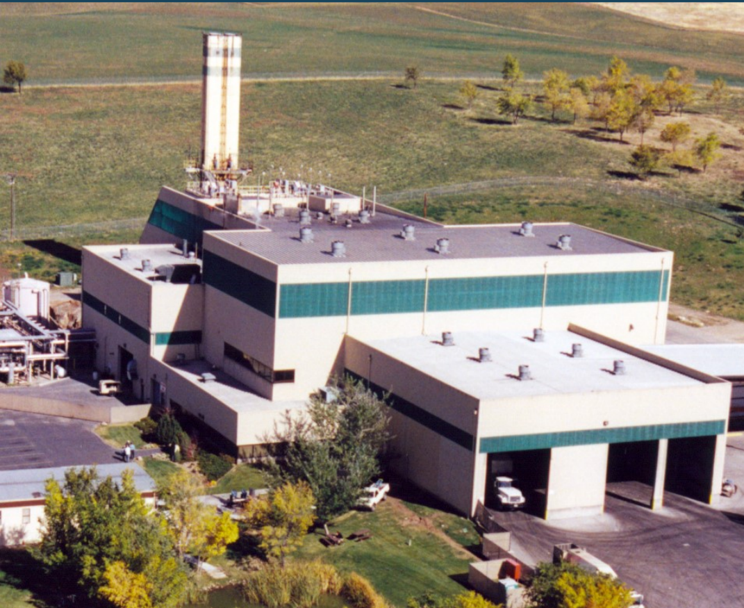
Wasatch WTE Facility prior to Deconstruction
