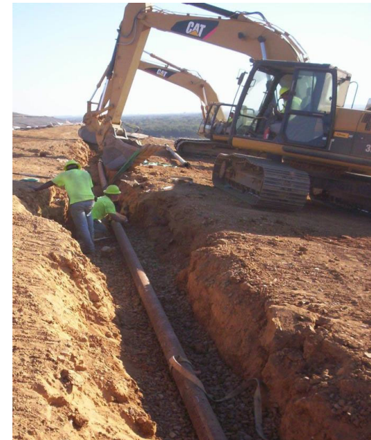
HORIZONTAL COLLECTOR DETAIL
