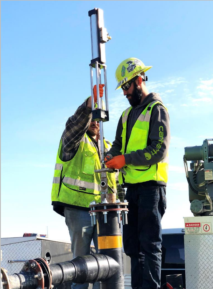
After piston rod lowered into downhole, attach it to drive rod of actuator
