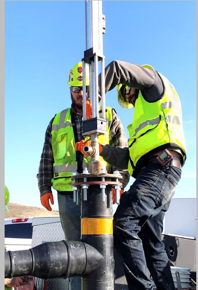
Secure pump/actuator onto wellhead
