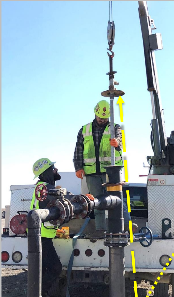
Wellhead assembly attached to final pipe section
