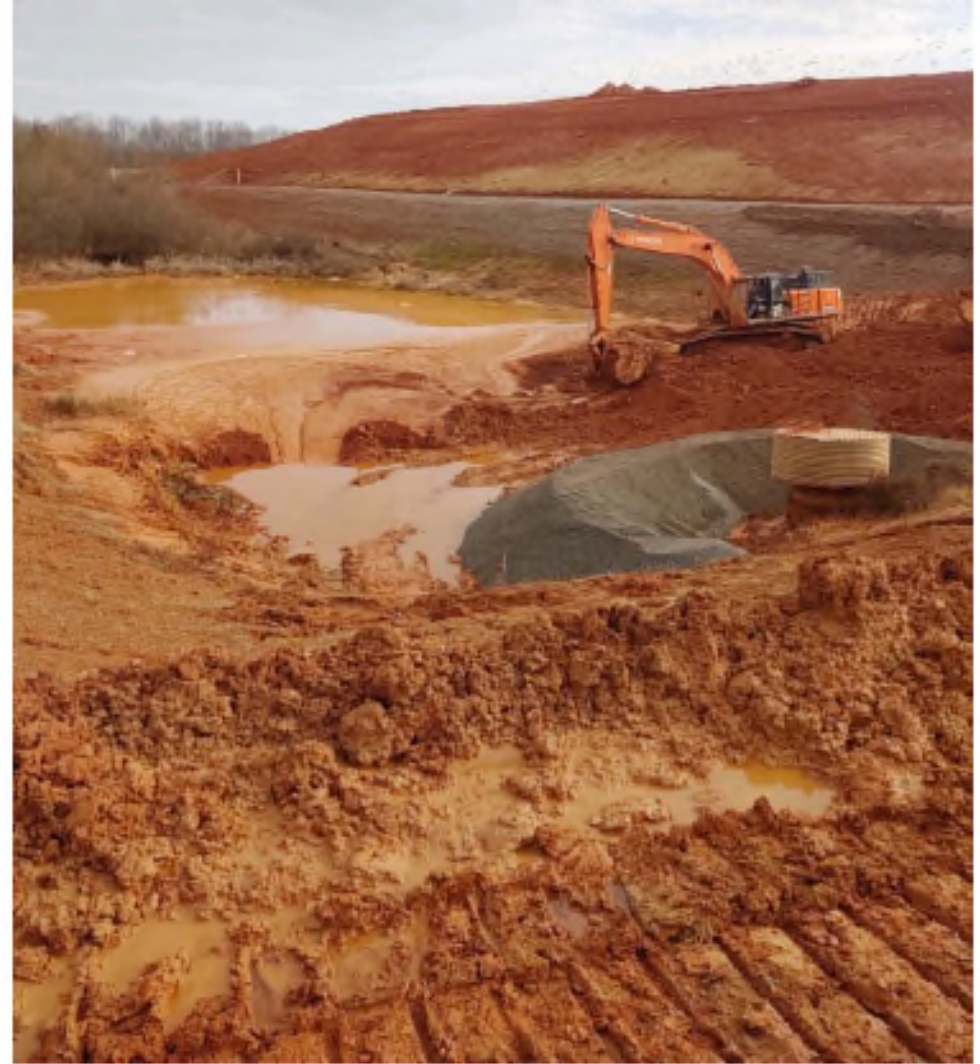
PHOTO 1: Pond cleaning and rock filter dam installation at sediment pond for Outfall 001
